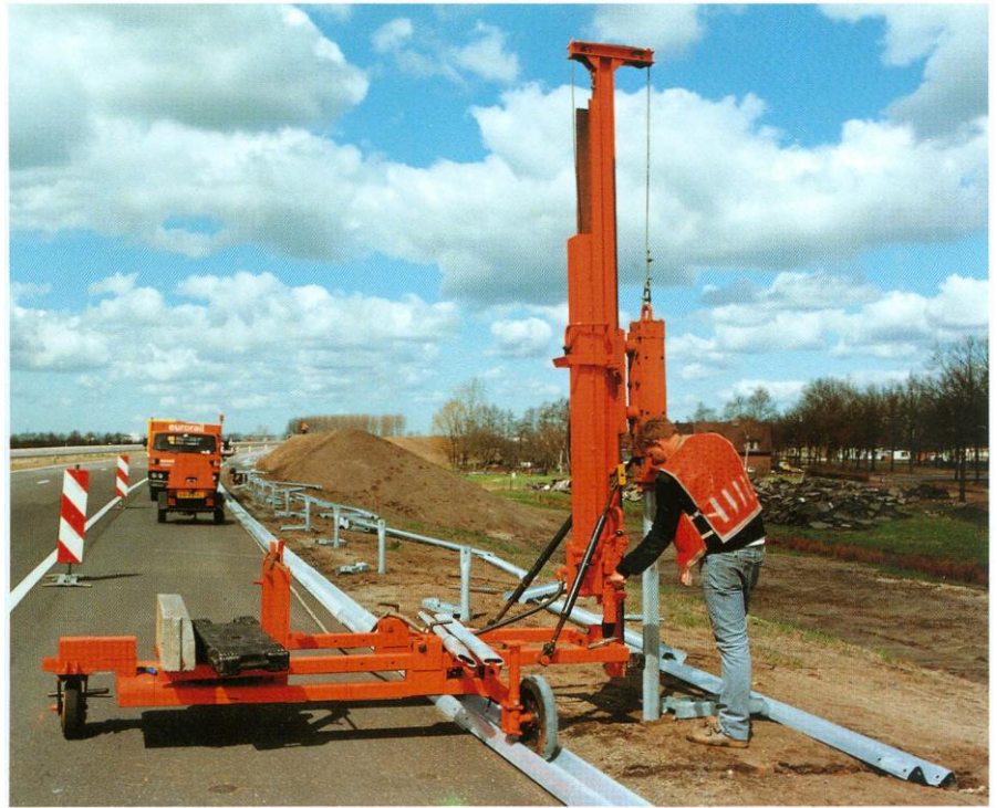
Guardrail-piledriver in action (type "Eurorail")
